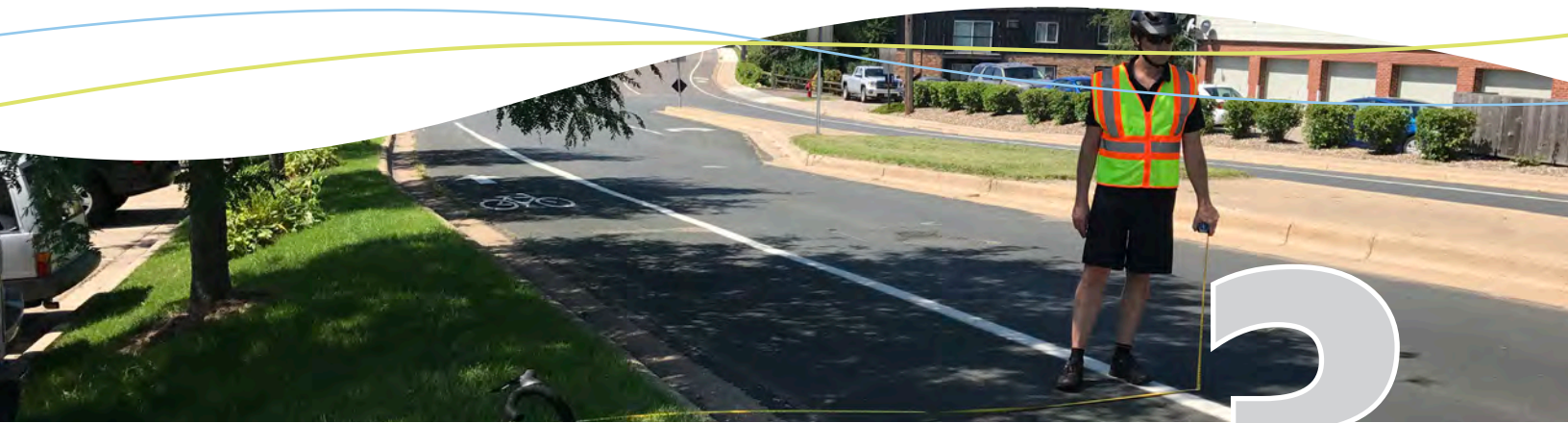
Park District staff conducting field work along segment A4 of the CPRRT | Edina, MN
